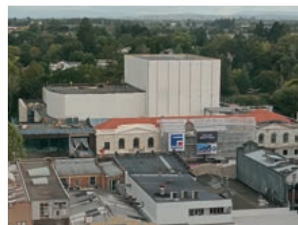
Waikato Regional Theatre under construction. Image Momentum Waikato
